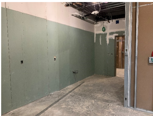
Level 1 Drywall in New Addition
